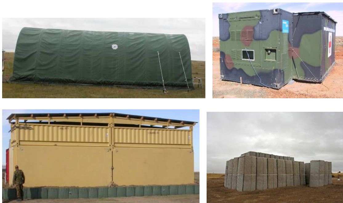
Figure 5. Examples of ES structures: tent, normal (ISO), heavily reinforced, HESCO
