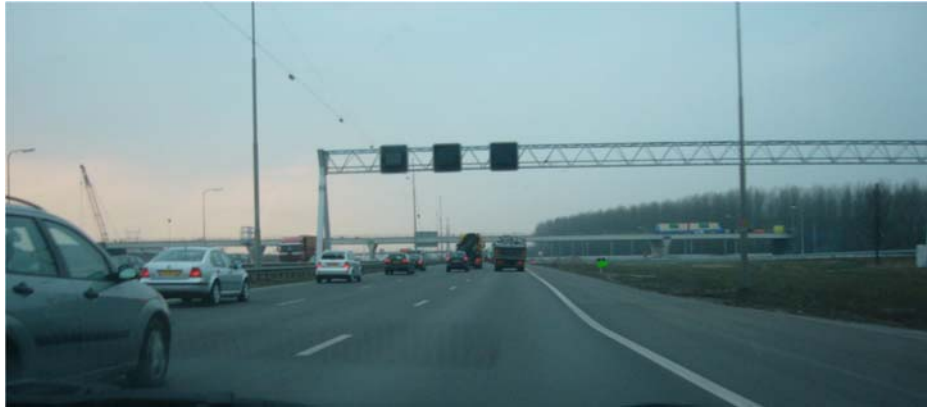
Figure 9 – Three-lane motorway toward location 2: change in horizontal alignment.
