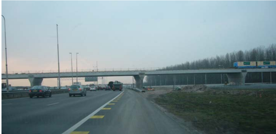
Figure 11 – Temporary exit for work-zone traffic on shoulder location 2.
