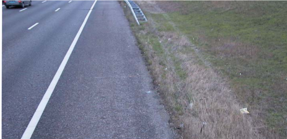
Figure 41 – Location 9, tracks behind guardrail.
