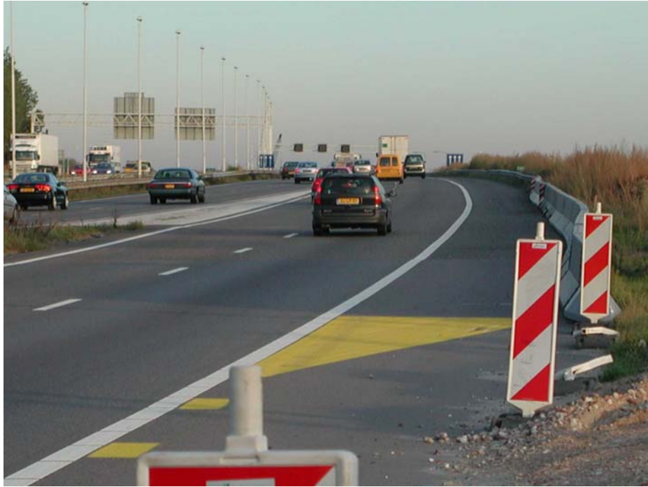
Figure 25 – Work traffic exit and barrier (behind last red/white pole), location 5.
