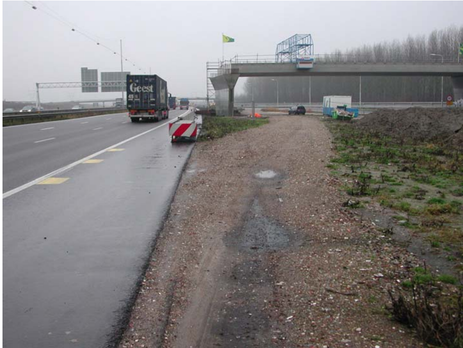
Figure 13 – Accident location 2 with old barrier at time of accident.
