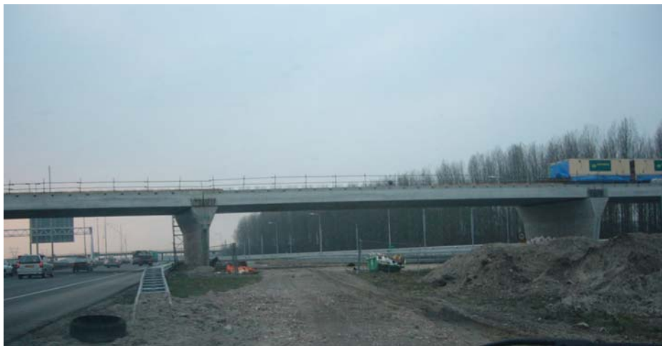
Figure 12 – Accident location 2 with new barrier at time of road-scene analysis.
