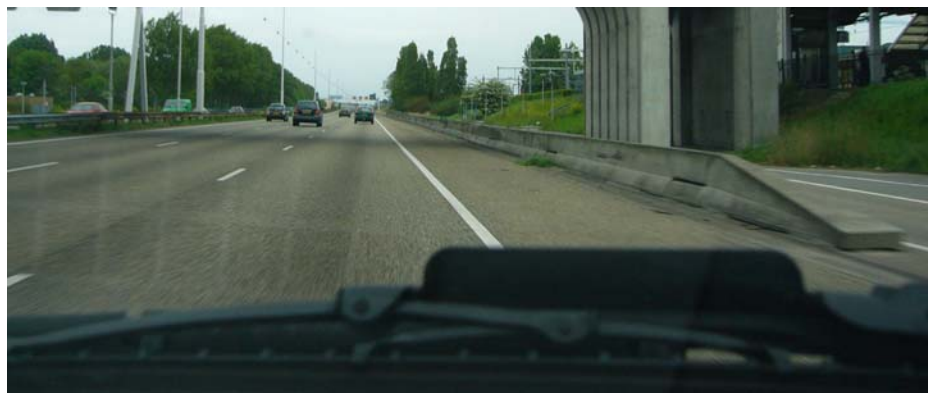
Figure 22 – View from motorway at barrier and pillar, location 4.
