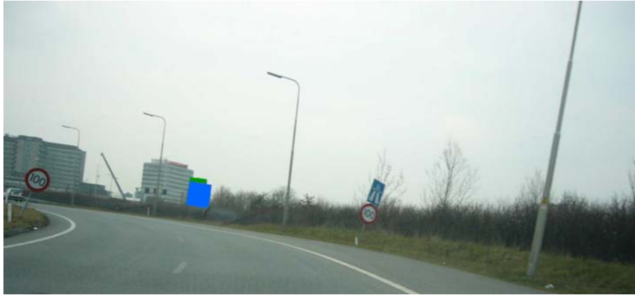
Figure 3 – Curve 1 at location 1 continued 2.
