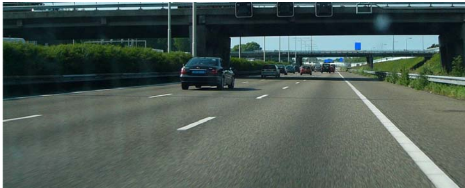
Figure 38 – Approach trajectory, location 9, before two viaducts (600 metres).
