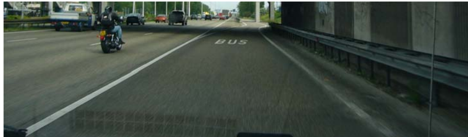
Figure 20 – Location 4 noise barrier (wall) and pillars of the crossover.
