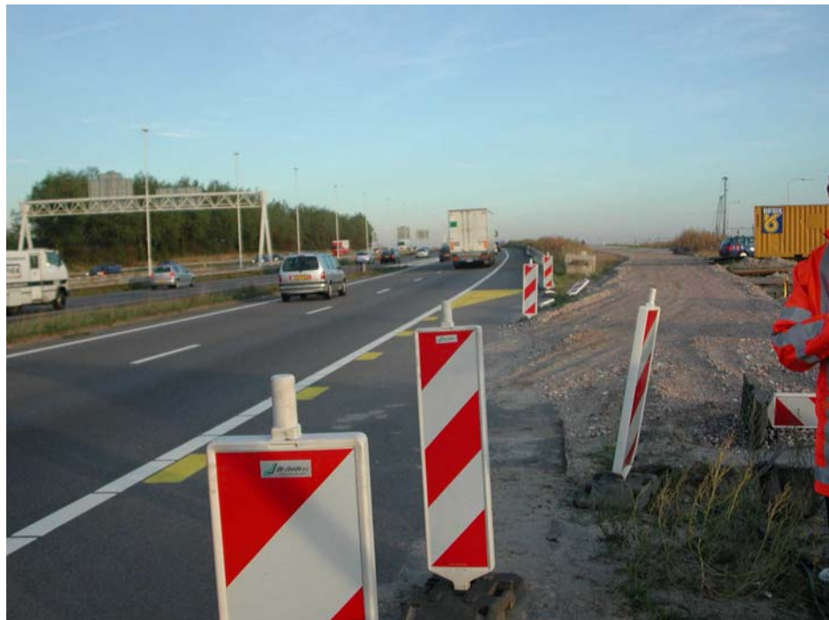
Figure 24 – Work traffic exit location 5.
