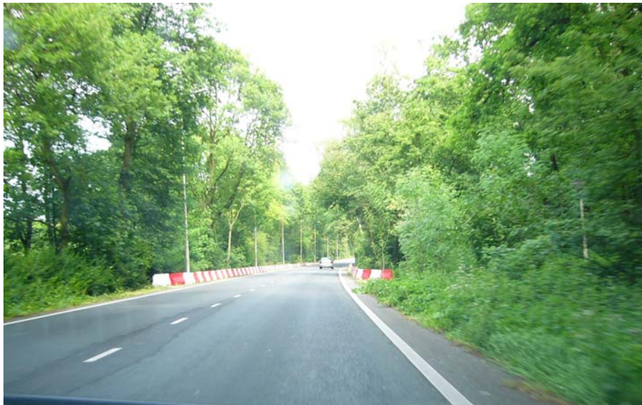
Figure 30 – Start of curve to the right of accident location 7: the red and white low plastic barrier is added after the accident.
