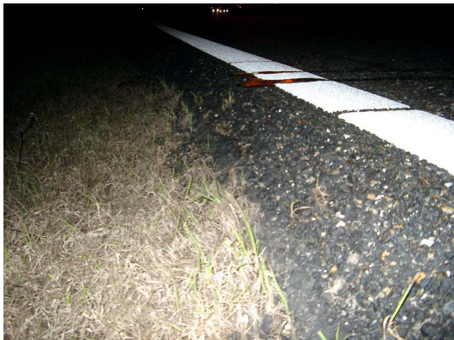
Figure 18 – Location 3 illustration of drop-off of roadside (b).
