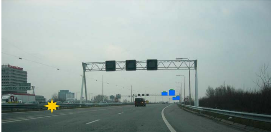
Figure 7 – Entrance of motorway with crash location (yellow star), location 1.
