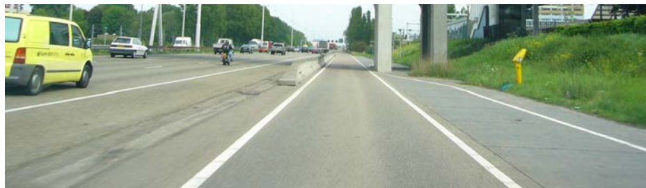
Figure 21 – Bus lane semi-separated by concrete barrier, location 4.
