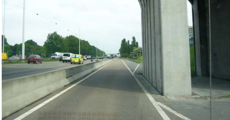
Figure 23 – Bus lane passing under crossover with unshielded pillar on right side, location 4.
