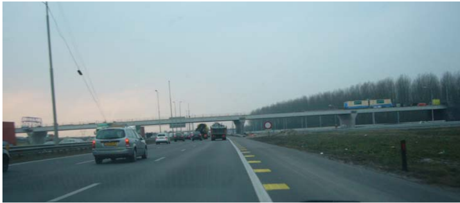
Figure 10 – Temporary exit lane for work-zone traffic indicated with yellow marking, location 2.
