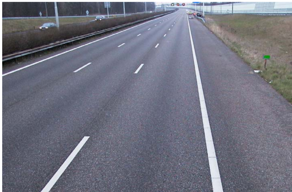
Figure 40 – Approach trajectory, location 9, halfway viaduct and end position vehicle.
