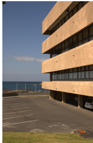
Figure 5: Balcony Parapets at IMT
