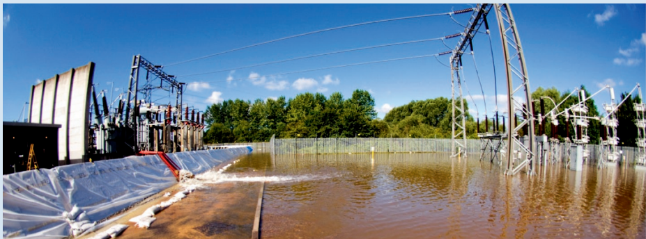
FIGURE 17: The Walham substation with a temporary flood barrier (photo: UK MOD Crown Copyright (2007))
