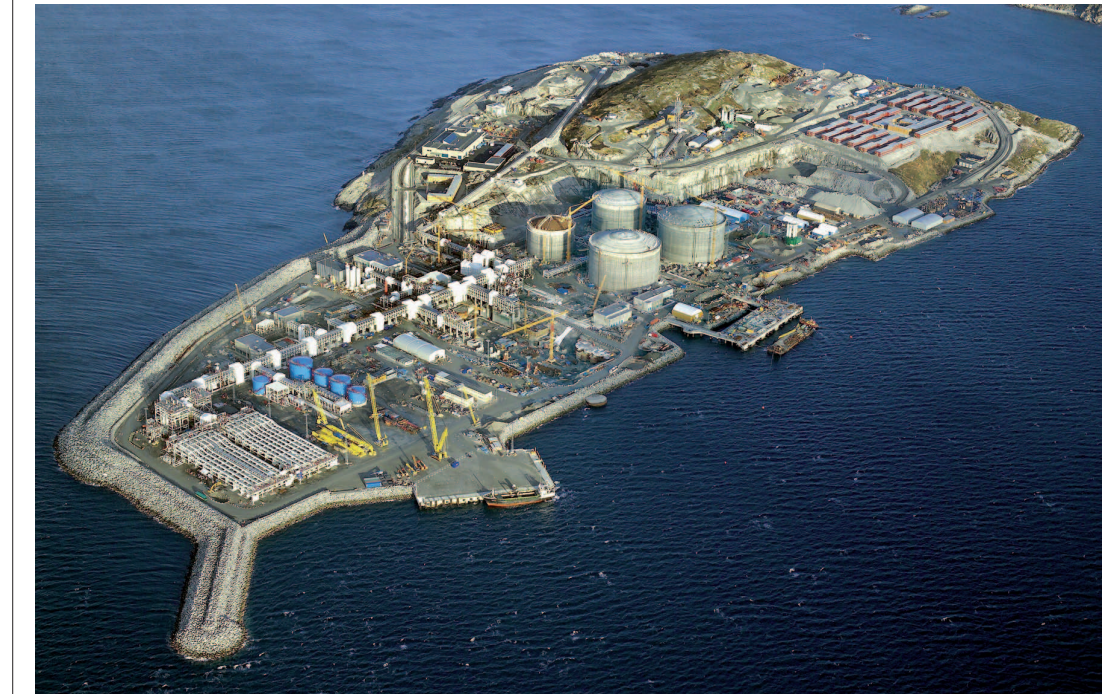
LNG liquefaction plant of Statoil at Snohvit
