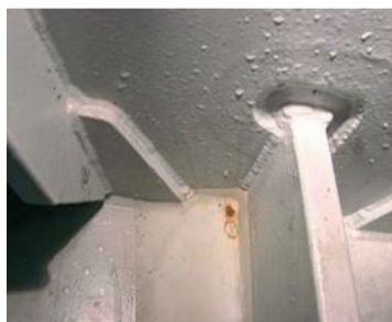
Fig 2. Example coating damage
