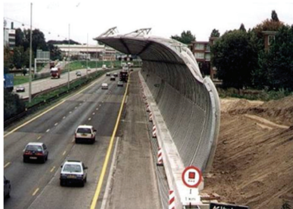
Figure 3: example of a road cover
