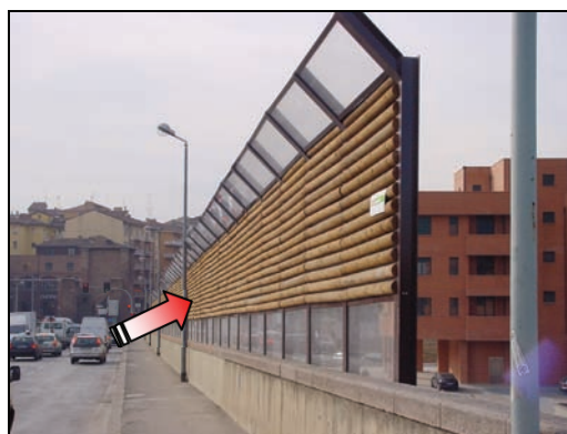
Figure 22: a noise barrier alongside a road (courtesy CIR Ambiente): the sound field (represented by the arrow) is not diffuse
