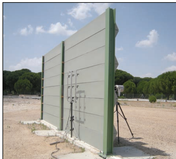
Figure 27: Sound insulation index measurements: sound source and microphone array near a sample noise barrier, in front of the acoustic elements
