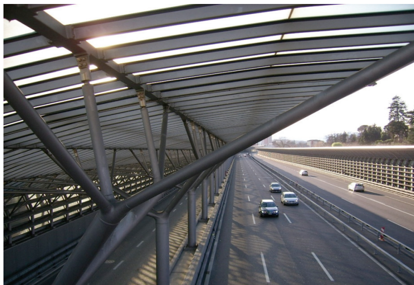
Figure 55: View of a transparent barrier / road cover near Lugano, Switzerland
