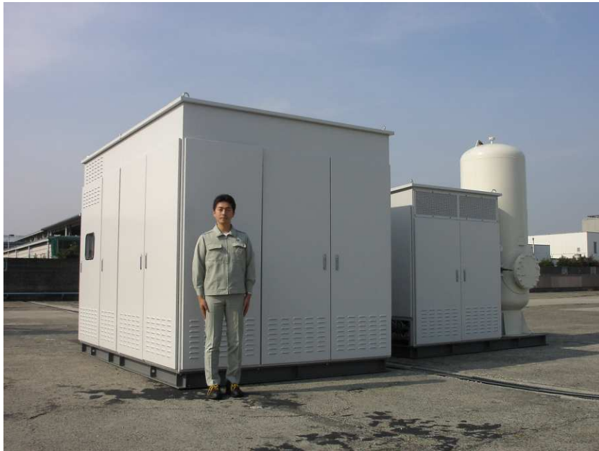
Figure 18: Compact reformer and compressor, 100 Nm 3 /h (source: Osaka Gas)
