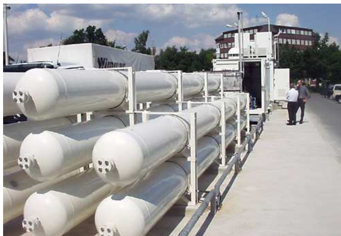
Figure 19: CGH2 Storage cylinders (35 MPa) in Hamburg (CUTE Project, source: http://www.h2stations.org/ )
